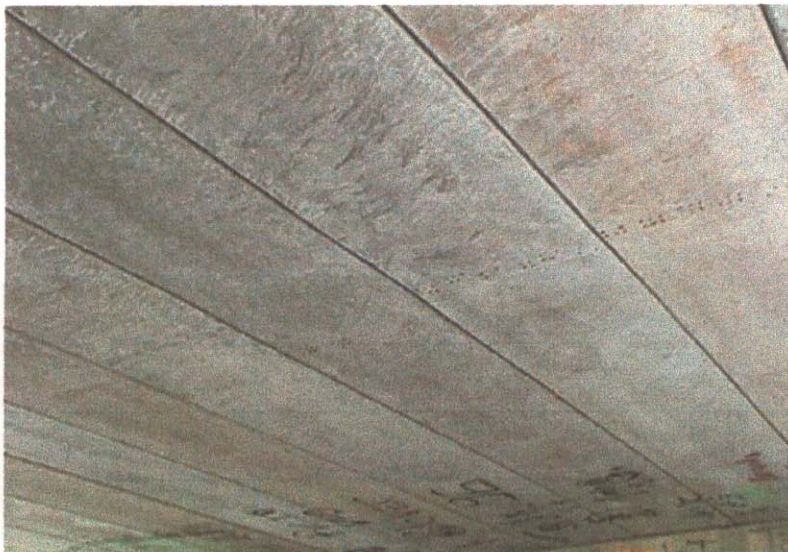
BOTTOM OF DECK
