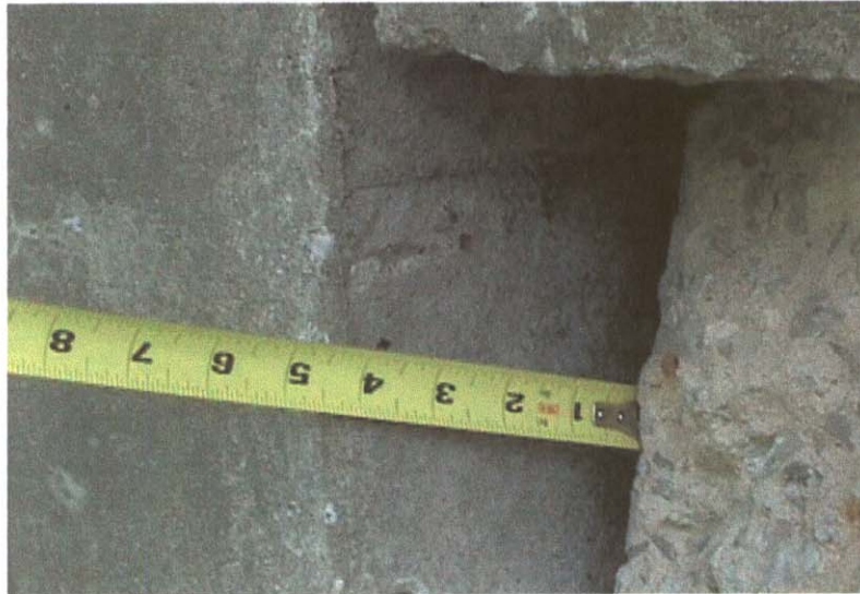
BREAKOUT ABUTMENT #1 BACKWALL RIGHT SIDE
